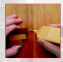
Filling ...and drop liquid filler into damaged area until area is slightly overfilled.
